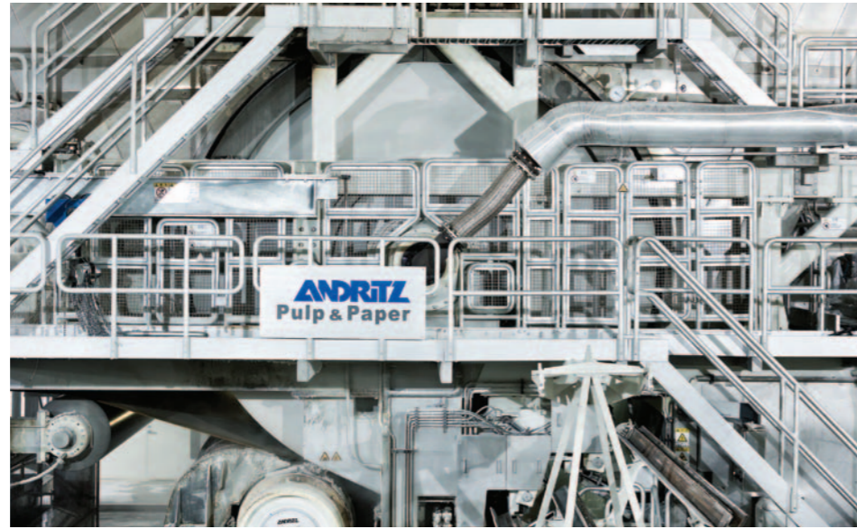
▲ The heart of the Hengan machines: 18 ft. diameter PrimeDry Steel Yankee.
