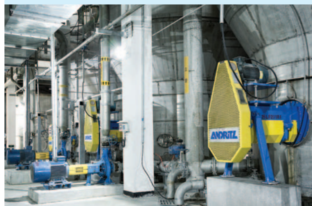
◀ ANDRITZ process pumps and agitators.
