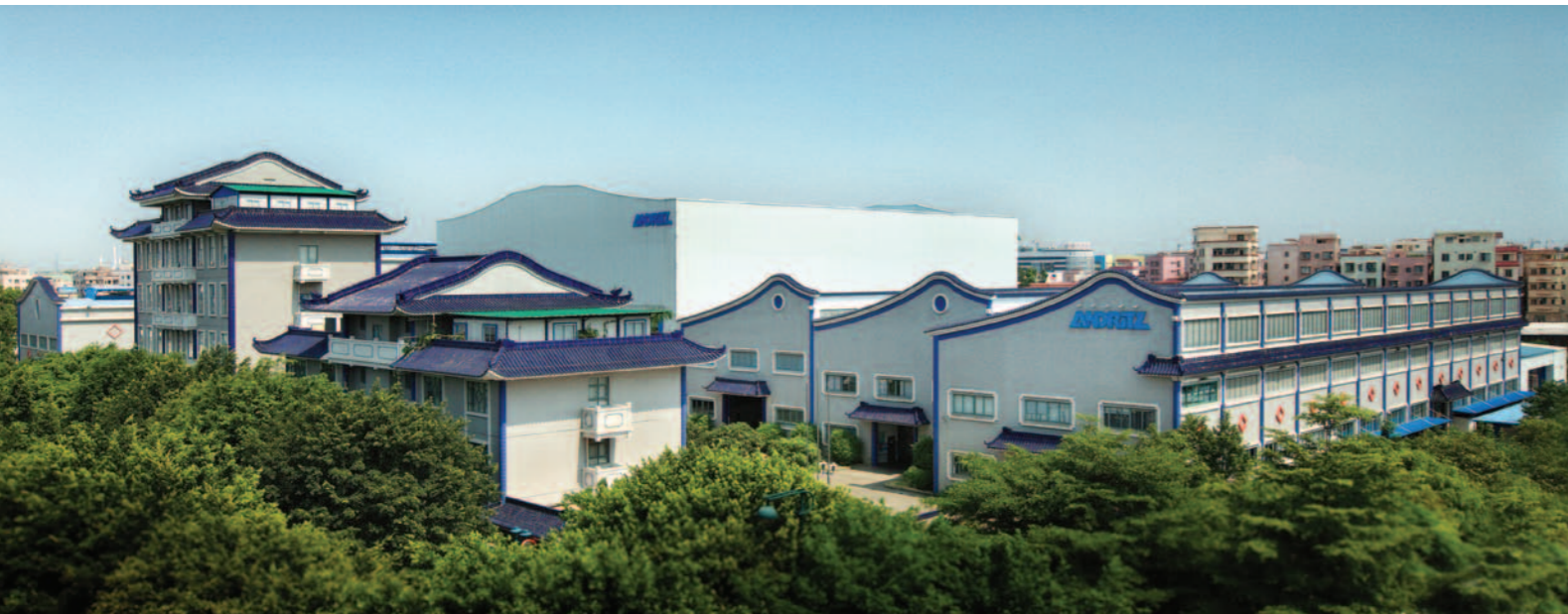
▲ Headquarter of ANDRITZ China in Foshan.
