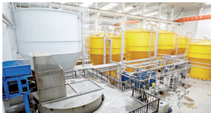
◀ Stock preparation plant delivered by ANDRITZ (pulper in the foreground).
