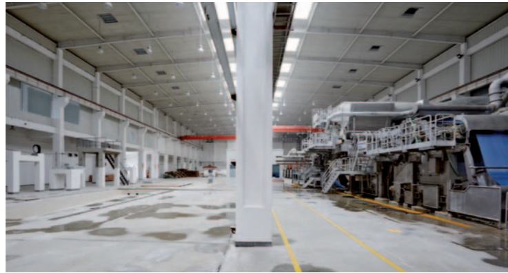
◀ TM1 on the right and the erection location for its twin, TM2, on the left. TM2 will start-up in 2015.
