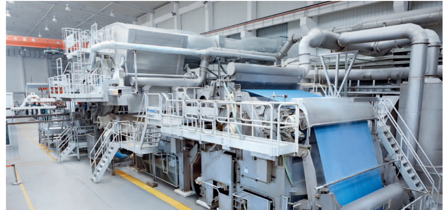
▲ The first one of the twins: PrimeLineCOMPACT TM1 at Hebei Yihoucheng, Baoding.
