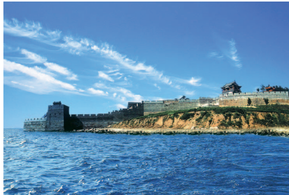
▲ A part of the Laolongtou Great Wall in Qinhuangdao City in Hebei province.
