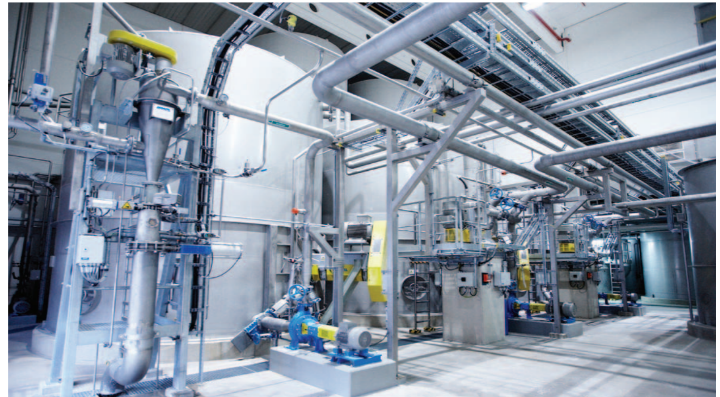
▲ As part of the package ANDRITZ delivered the stock preparation system for virgin fibers, a broke processing line, and the systems for water recirculation and fiber recovery.
